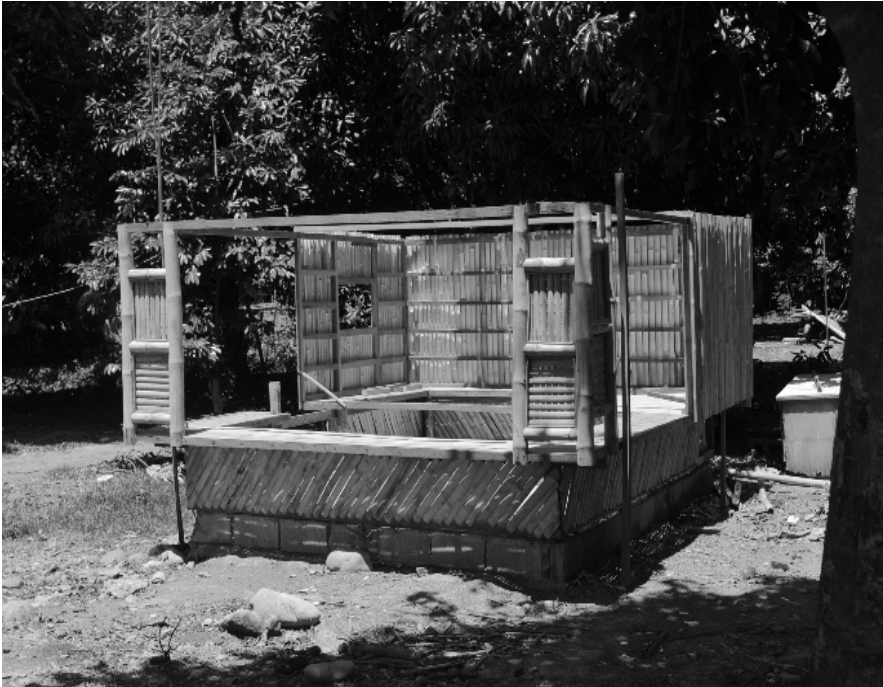
Figure 5. A nipa hut ( bahay kubo ) work-in-progress.
