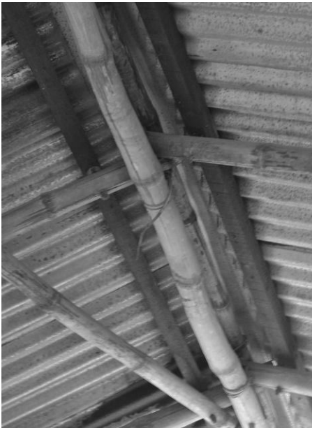
Figure 2. Kawayáng bayog as a roof support.
