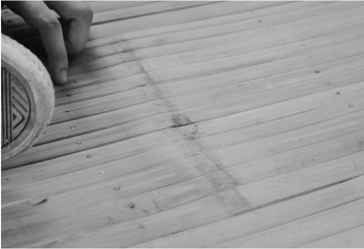
Figure 15. “Eye” of the bamboo on slats at the floor of a nipa hut.
